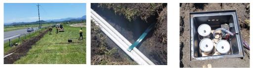
A bilge pump with float-valve switch was installed at the base of the pit to remove water to the Council drain outside the track. The pit was then covered with a metal grate, plastic sheeting, and geotextile cloth to protect the gauges. Lastly, the pit was covered with soil and the turf left to regenerate.
