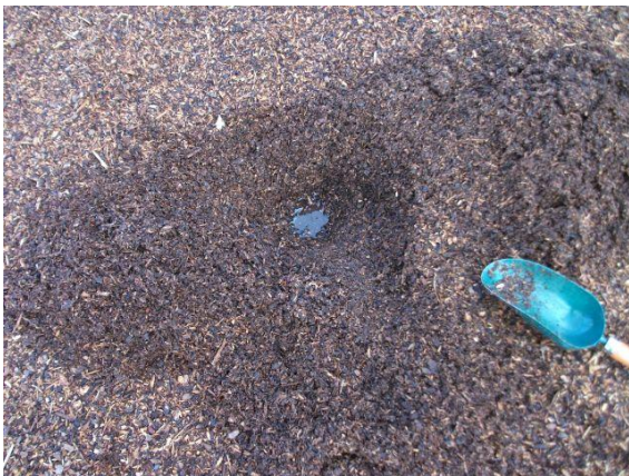
Figure 13a. A shallow hole under the swings area that had not been drained shows free water just below the surface.
