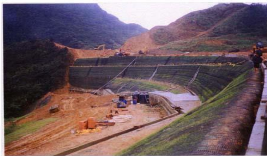
RETAINING WALL OF "JAWULOOM" HIGHWAY 西溪公路大武仑段加劲挡土墙
